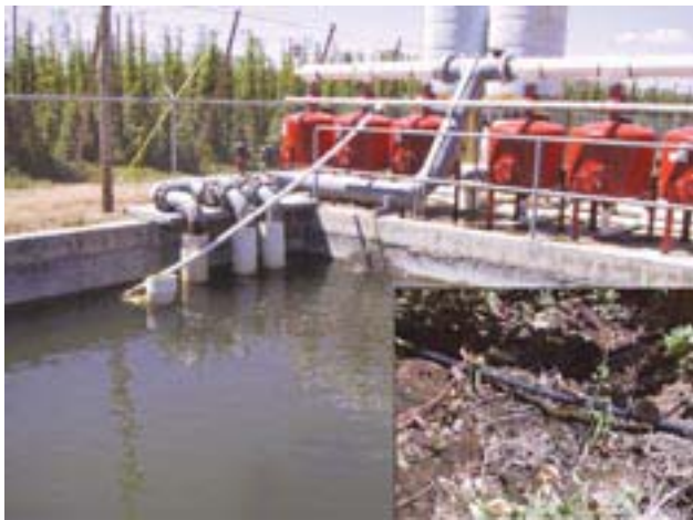
Drip irrigation system with buried line.
