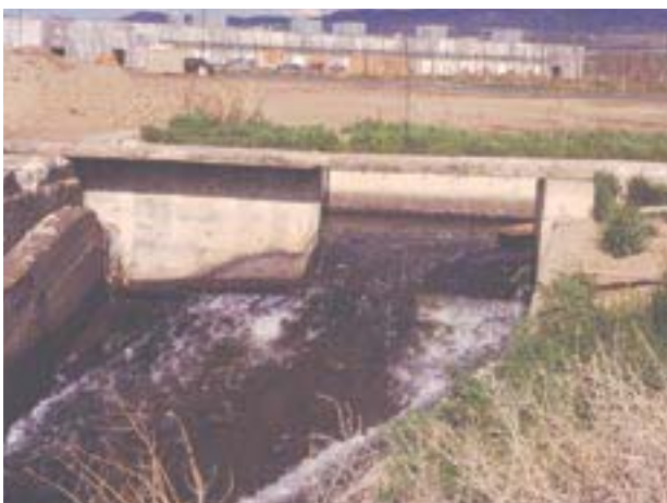
In plentiful water-supply years, some irrigation water is spilled directly into agricultural drains.
