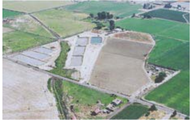
The Roza-Sunnyside Board of Joint Control routes agricultural-return flow into two separate networks of inter-connected ponds (constructed wetland) to reduce sediment and nutrients in Yakima River.
