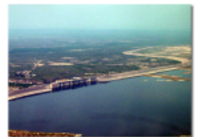
AMISTAD DAM - AERIAL VIEW
