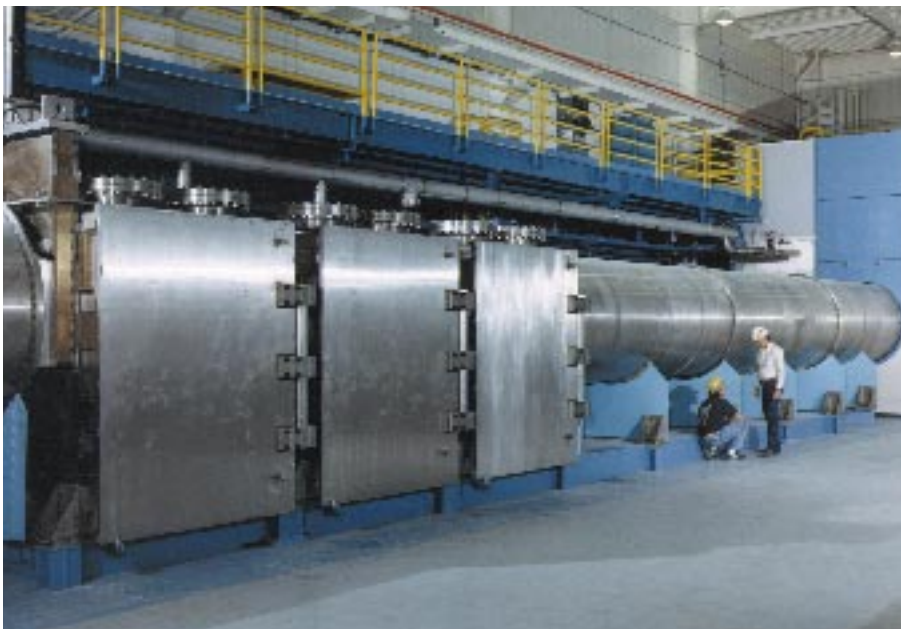
The separator demonstration facility at Lawrence Livermore's laser isotope separation (LIS) pilot plant tested full-scale equipment. One of three separator units shown for enriching uranium was operational for demonstrations. Also visible are beam tubes for transporting precisely tuned laser light to the separator units.
