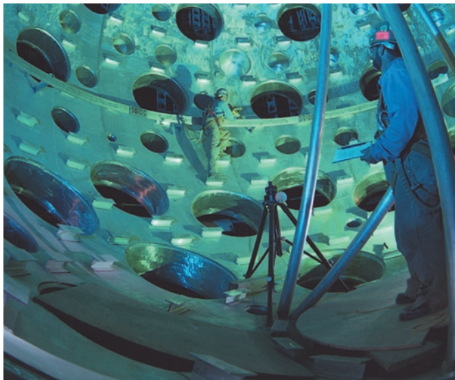
The 10-meter-diameter target chamber of the National Ignition Facility was assembled from 18, 10-centimeter-thick aluminum sections. It is located in a 7-story target bay, weighs about 450,000 kilograms, and has been precision aligned to better than 1-millimeter accuracy.
