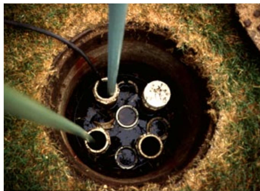
Figure 3. A look down an Orange County Water District monitoring well.
