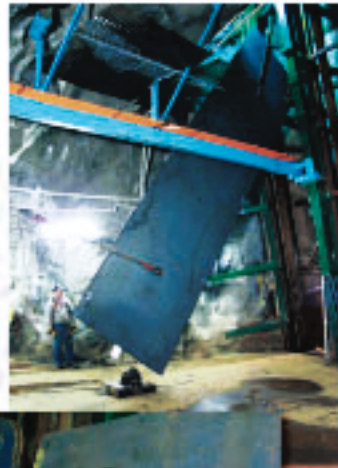
Steel plates 2 by 8 meters are lowered down the mine shaft.
