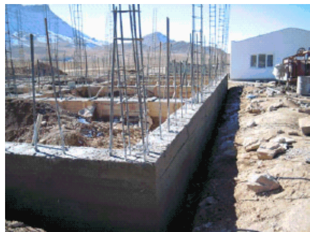
Foundation and wall construction of a new school.
