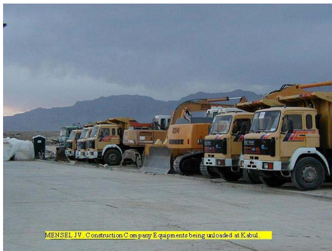
Equipment for Afghan Highway Section C, KM 92 – KM 177, June 2003
