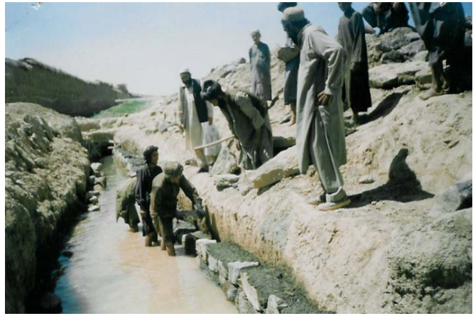
Rehabilitation of irrigation system using cash-for-work labor, Spring 2003
