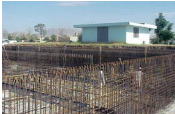
USAID constructed this storage reservoir to improve water supply in Kandahar.
