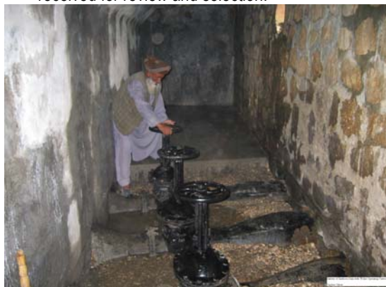
Worker Operating Valves in Repaired Gallery of Sar-e-Haus Dam
