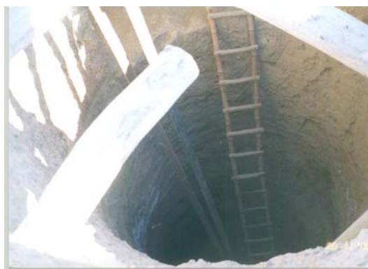
Entrance to karez: Afghan laborers descend into underground tunnels like this one to clean accumulated silt and make repairs.
