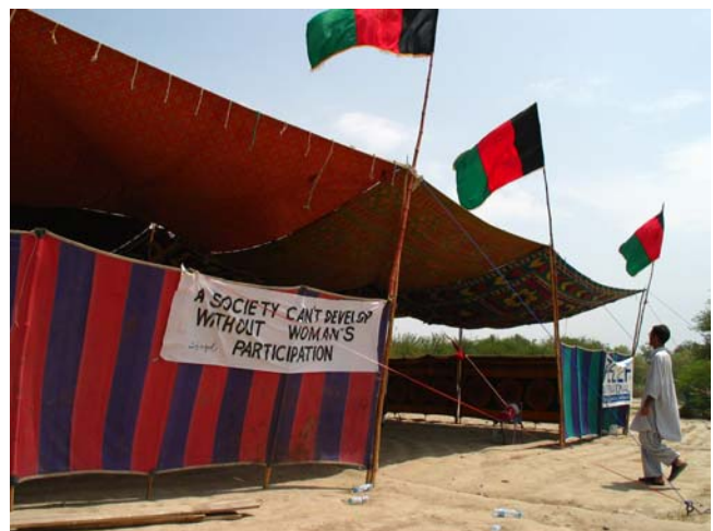
Groundbreaking ceremony for the construction of a women's center in Jalalabad on August 3. USAID/Kabul Mission Director and the Deputy Governor of Nangarhar Province attended the event held in the tent, above, festooned with flags of the Afghan central government.
