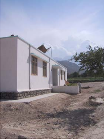
Pierakhil village, Khogyani district, Nangarhar: Pierakhil Primary School
