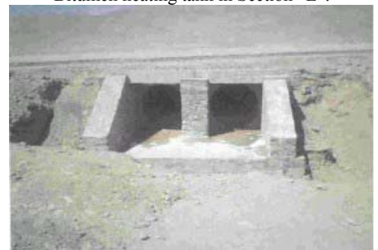
Stone masonry culverts in Section "B".
