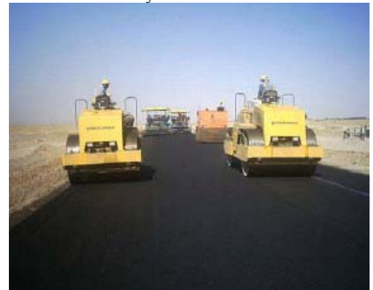
Rolling newly-laid ATB in Section "D".
