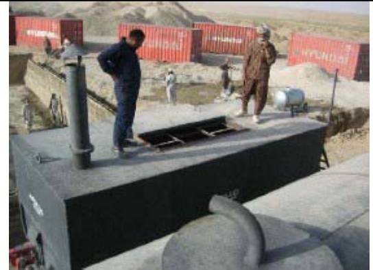
Bitumen heating tank in Section "E".
