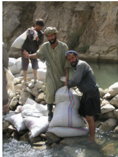
Local Afghans earn wages rebuilding irrigation infrastructure in their community.
