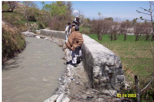
Strengthened canal walls increased irrigation in Khogyani District, Nangarhar.
