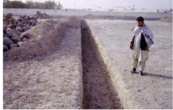
Excavation for the foundation of Saeed Mortza School in Ghazni province.
