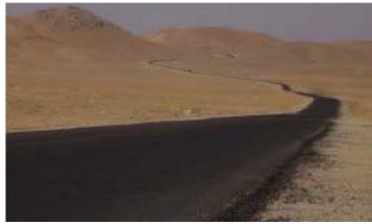
Newly laid asphalt treated road base near Ghazni..
