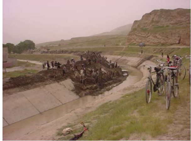
Afghans working on the Gawargan Canal. Photo credit: Development Alternatives, Inc.
