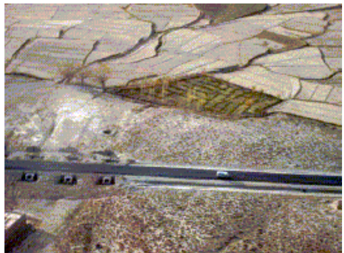
A section of the newly paved Kabul-Kandahar Highway.
