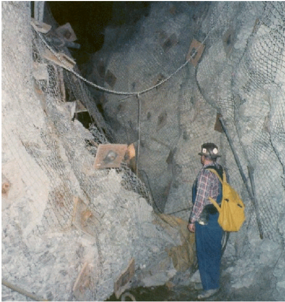
Area extensively damaged by rock burst in hard-rock mine.
