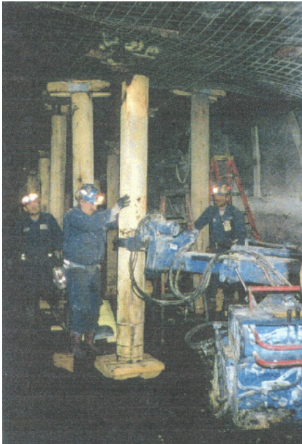
Installation of novel roof support system with hydraulically powered lifting device.
