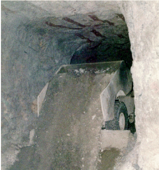
Truck depositing backfill in mine.
