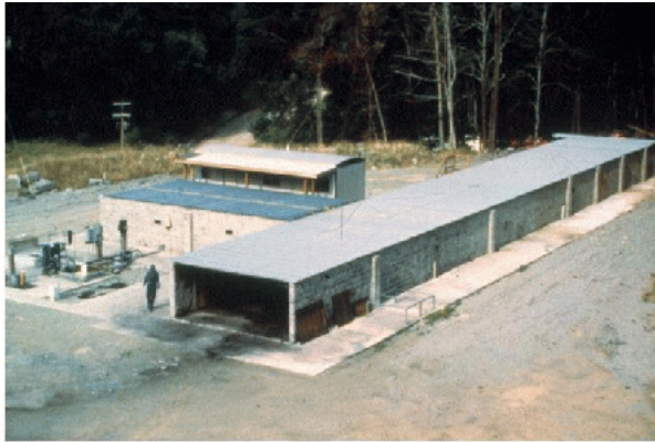
Fire suppression facility at Lake Lynn Laboratory.
