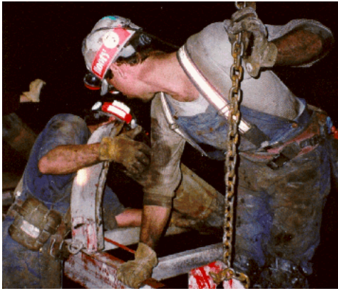
Removing conveyor belt in an underground mine.
