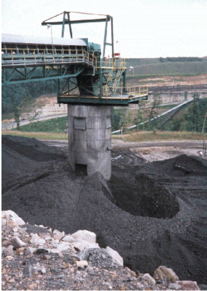
Void created in surge pile.
