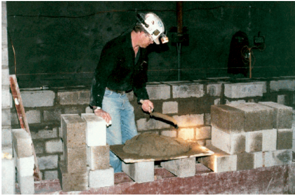
Construction of standard seal.
