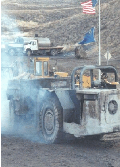
Diesel fumes generated by mining machines.
