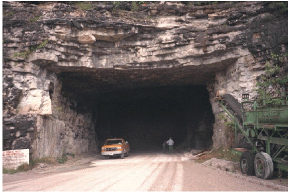
Underground limestone mine portal.
