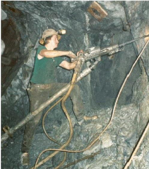
A lighter jackleg drill could reduce injuries among drill operators.
