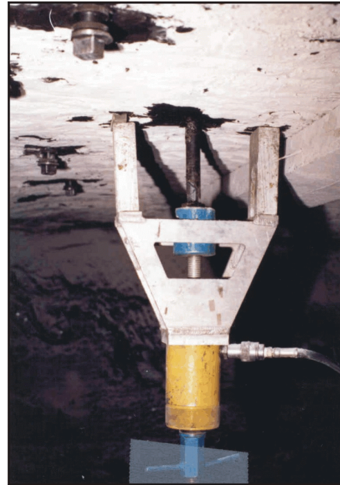
Figure 4.—A smooth hole lowers anchorage strength, as seen with this bolt as it pulls out of the hole.
