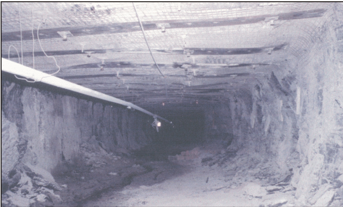
Figure 8.—Surface control in the form of a "Monster Mat" installed with cable bolts.
