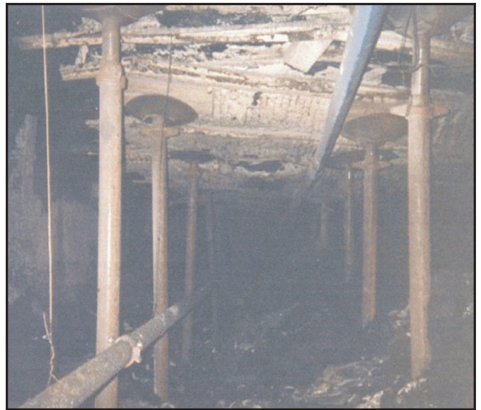
Figure 13b.—Inby area supported by ACS supports.
