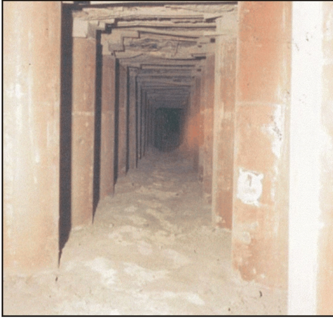
Figure 14a.—Outby area supported by Burrell Can support.
