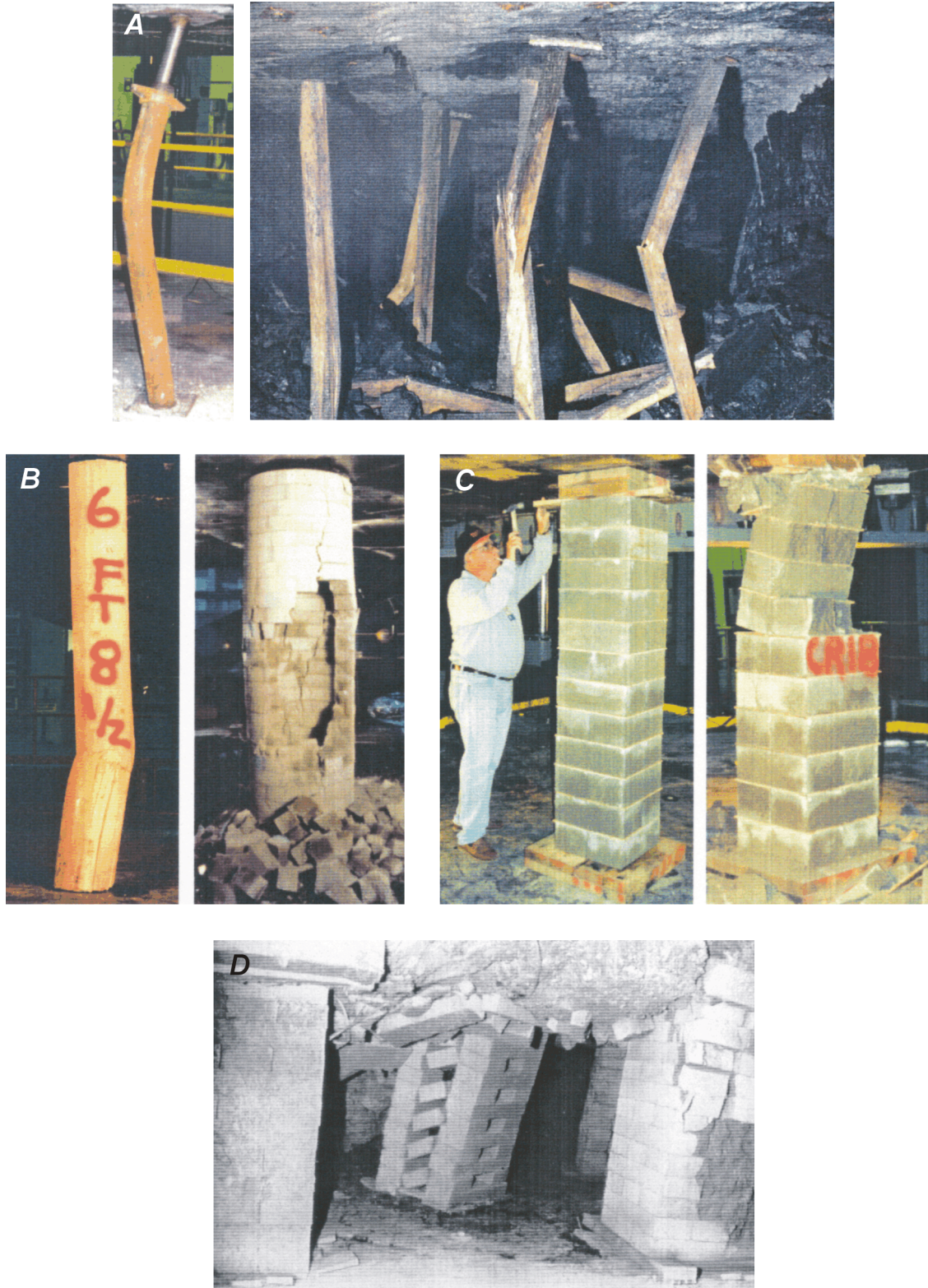
Figure 24.—Examples of support instability. A, buckling; B, material failure; C, eccentric loading; D, lateral roof-to-floor movement.
