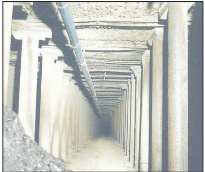
Figure 12a.—Outby area supported by Propsetter support.
