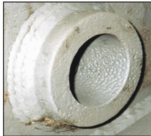
Figure 8.—Corrosion of a lemniscate link clevis.
