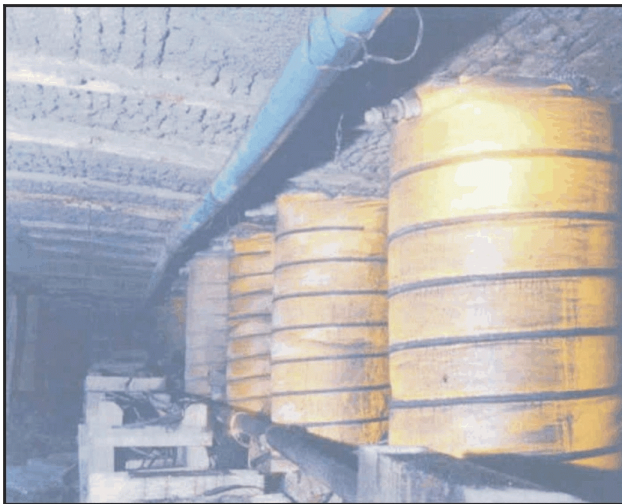
Figure 11b.—Inby area supported by pumpable crib.
