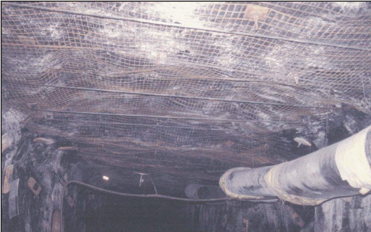
Figure 26.—Cable trusses installed in the headgate entry.
