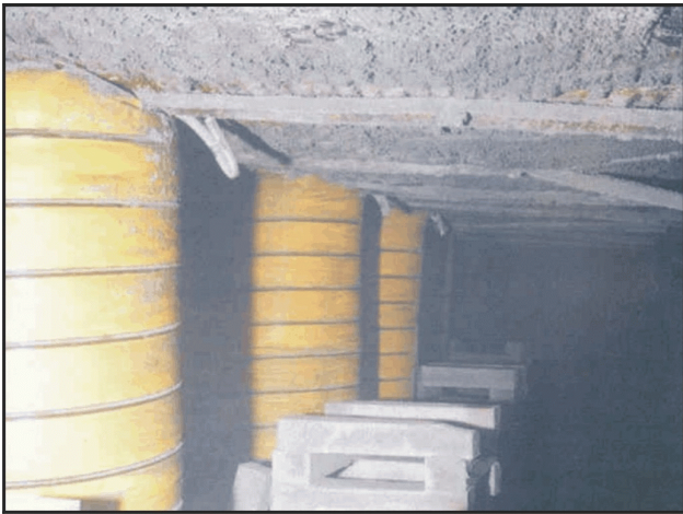
Figure 11a.—Outby area supported with pumpable crib.
