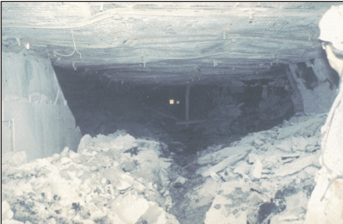
Figure 17.—Tailgate behind the shields kept open with cable bolts.
