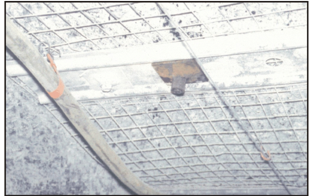
Figure 3.—Cable bolt system installed in a tailgate.
