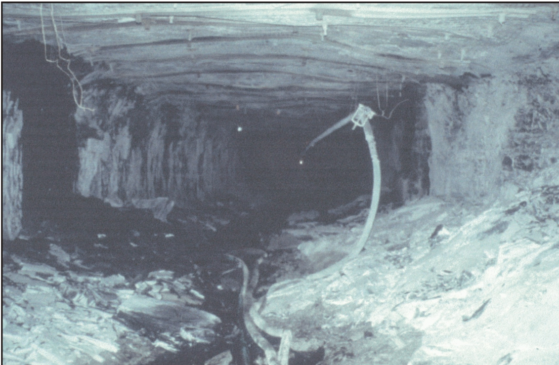
Figure 14.—Tailgate abutment zone outby the face supported with cable bolts.
