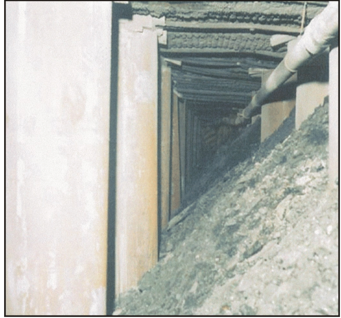
Figure 14b.—Inby area supported by the Burrell Can support.
