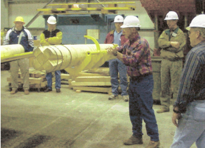
Figure 17. —Apparatus used for setting timber posts. (Photo courtesy of Strata Products USA).
