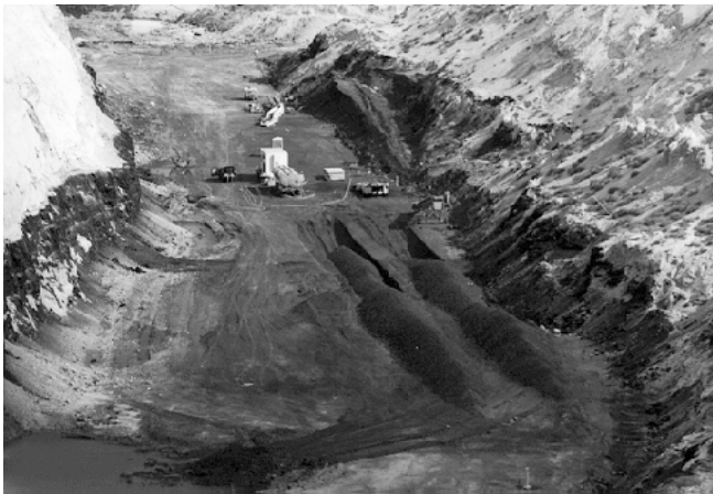
Figure 10.—Two 90-m cuts.
