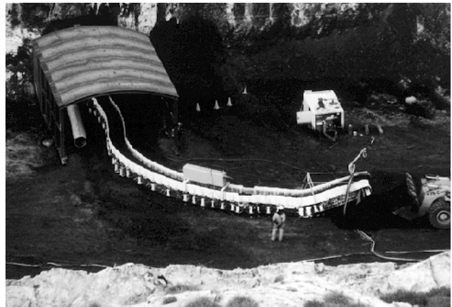
Figure 12.—Haulage system.
