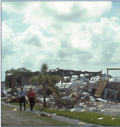
Hurricane damage devastates a community.
