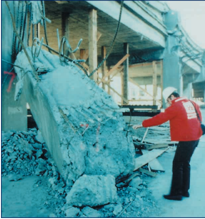
Well-trained Public Assistance inspector examines earthquake structural damage to Oakland overpass.
