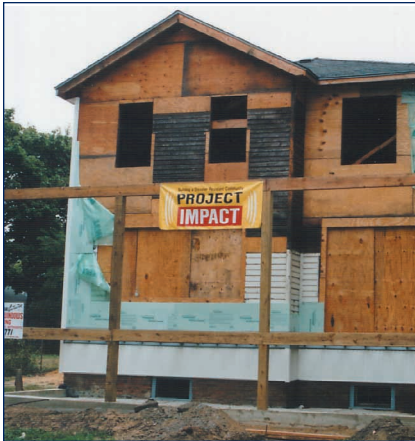
A home in Project Impact community Freeport, New York is being retrofitted with hurricane-resistant measures.
