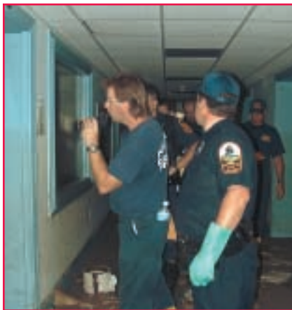
Re-entry crews inspect each home and business for contamination and structural integrity before occupants are allowed to return. FEMA NEWS PHOTO BY LIZ ROLL
