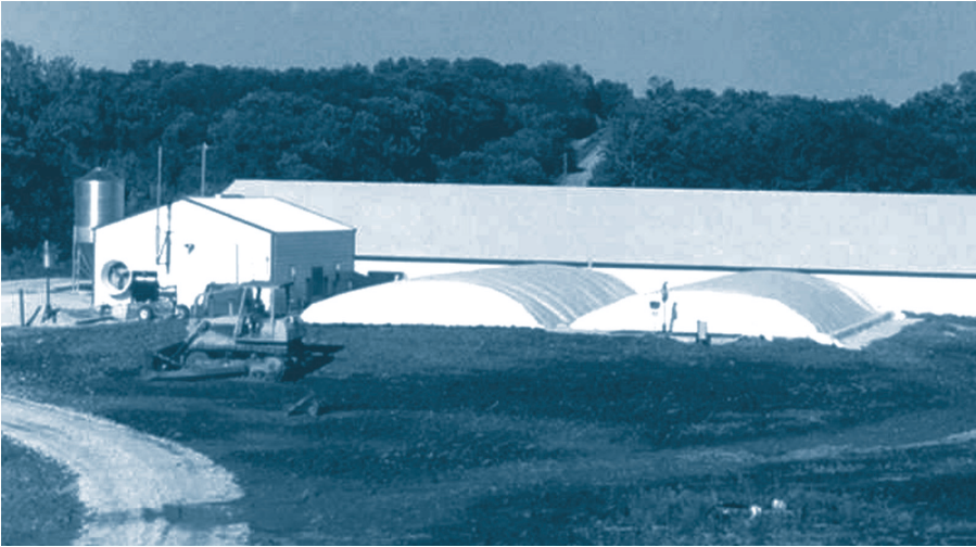
Complete mix digester.
