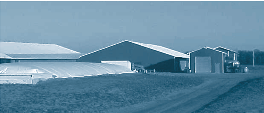
Plug flow digester.
