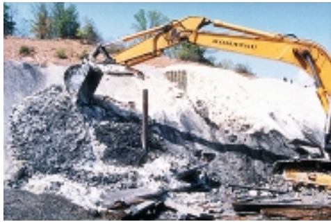
Smelter wastes containing up to 12% arsenic near Bunker Hill have been removed to a safe containment facility.
