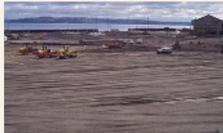
Cleanup in progress
