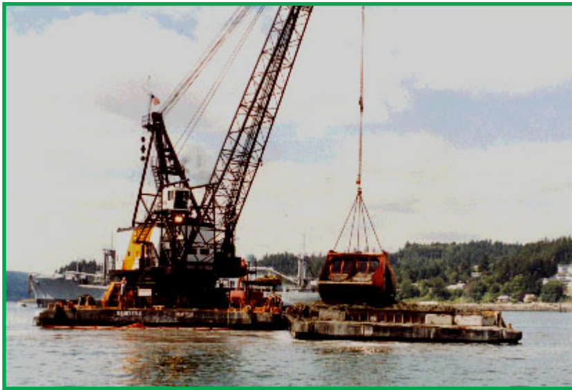
Dredging of PCB contaminated sediments in Sinclair Inlet.
