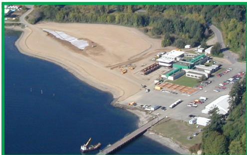
Crews finish placing new sand and cap over old dump.
