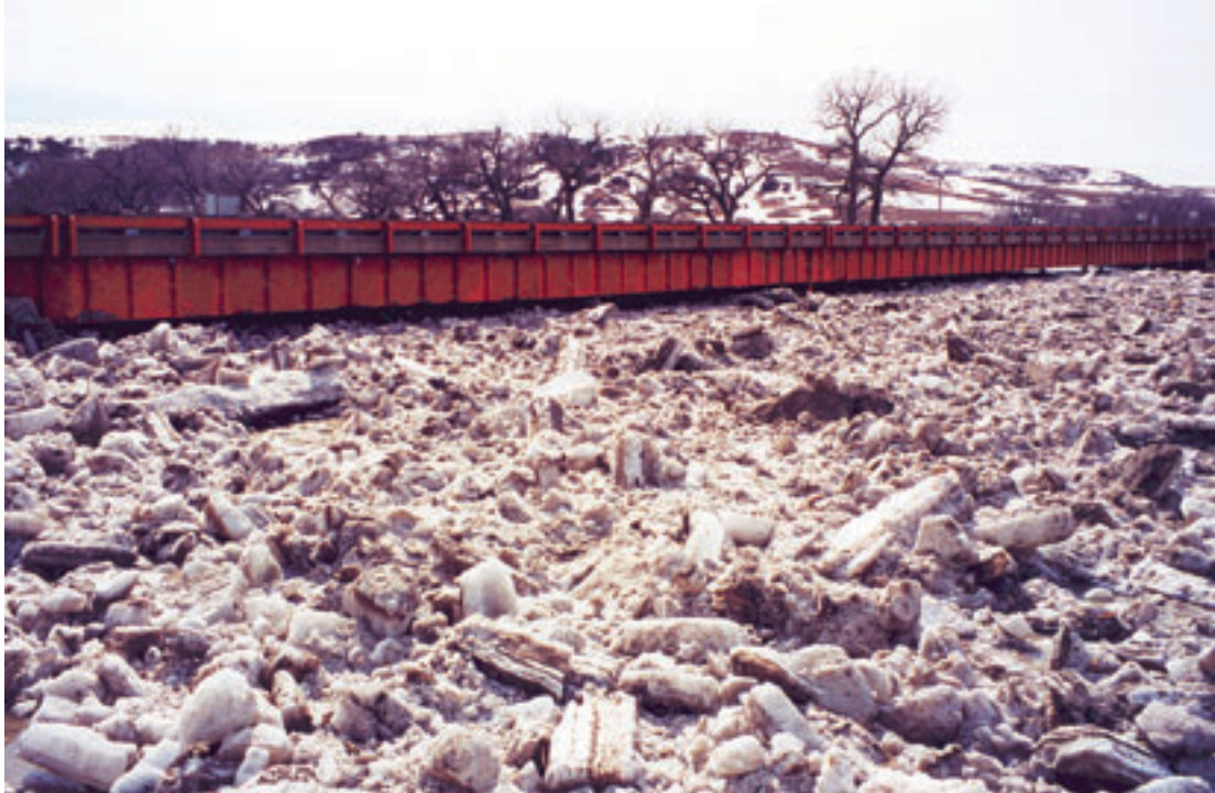
A Ice jam (no movement of ice) looking upstream of bridge
