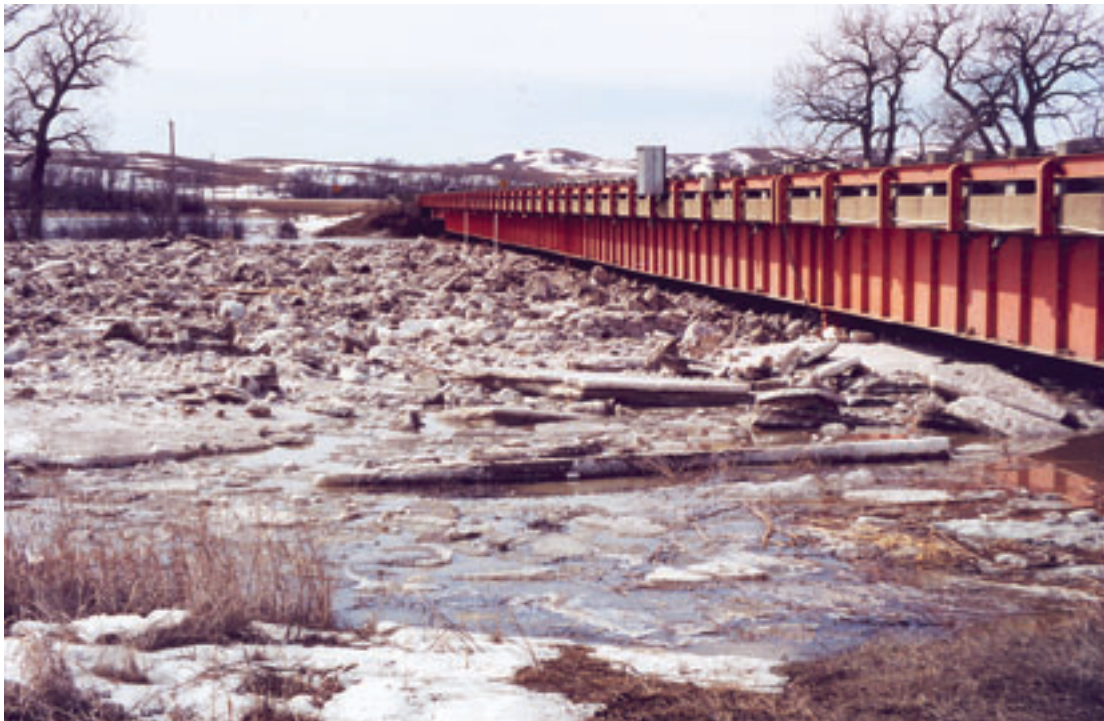
B Ice breakup downstream of bridge with flowing ice
