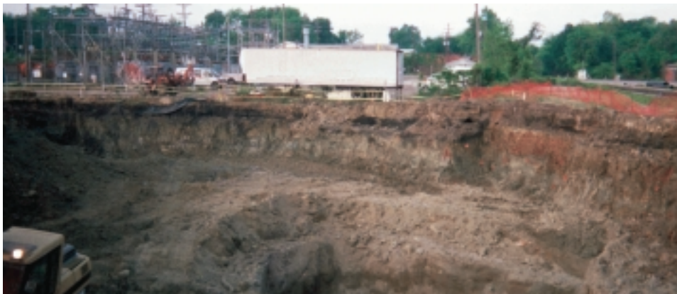
After tank removal.
