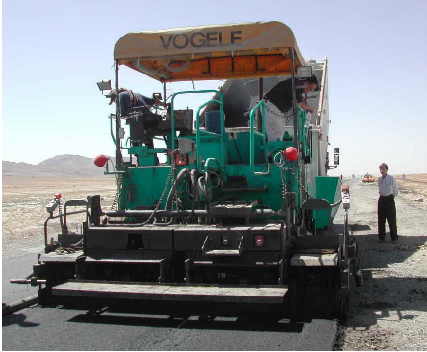
A photograph of a RIG/Manila auditor observing a subcontractor applying asphalt. This photograph was taken in August 2003 about 50 kilometers west of Kabul, Afghanistan.
