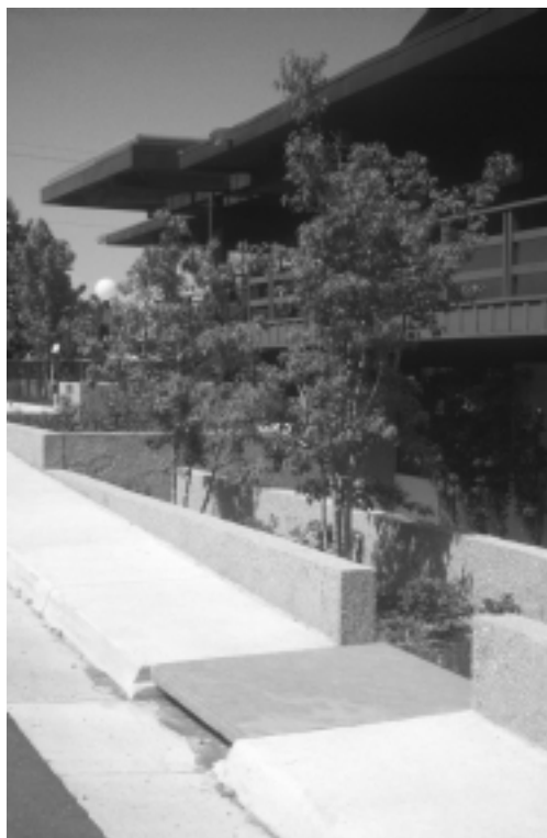
Runoff flows under sidewalk into gardens around the building.
