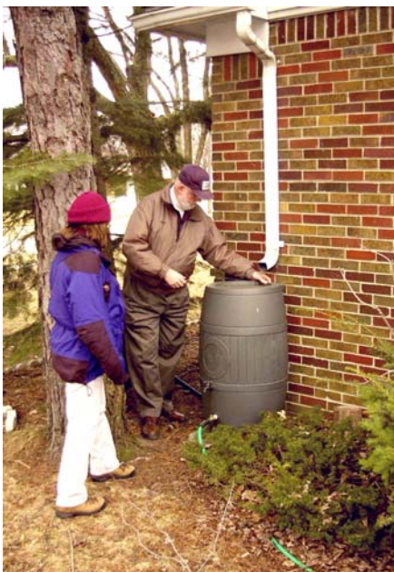
Installing a rainbarrel at a roof downspout
