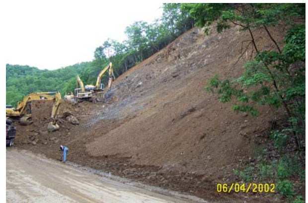
Heavy equipment clears the slide material to prepare for compost application.
