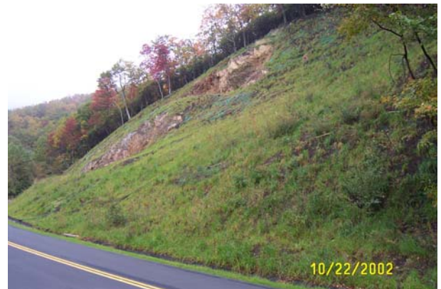
Vegetation was reestablished on the slope within 5 months of the slide.
