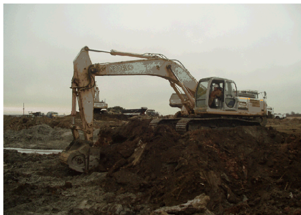
Excavation in Low Fill Area
