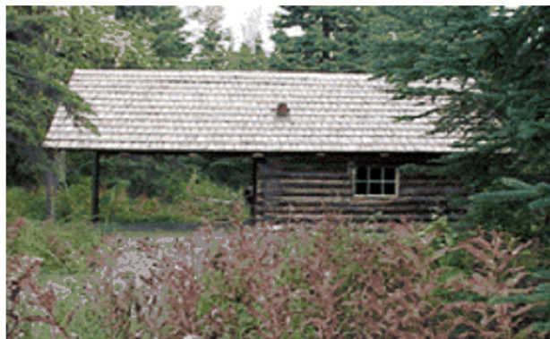
Restored Cabin at Kenai NWR Visitor Center - Soldotna, Alaska
