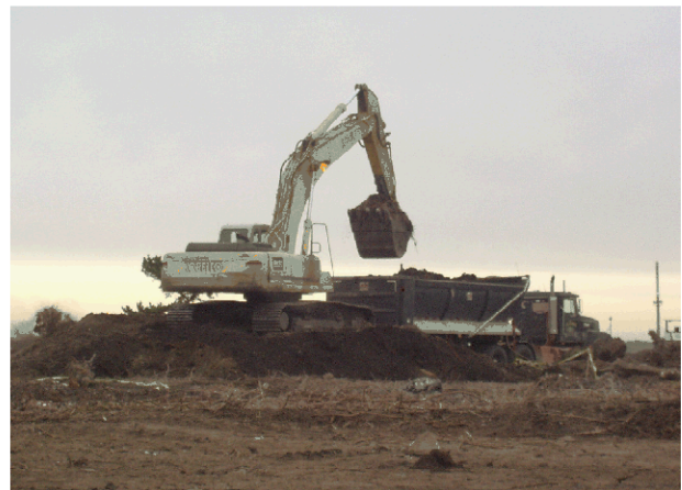
Loading Lead-Contaminated Soil
