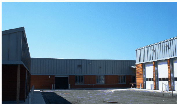
South View into Maintenance Complex
