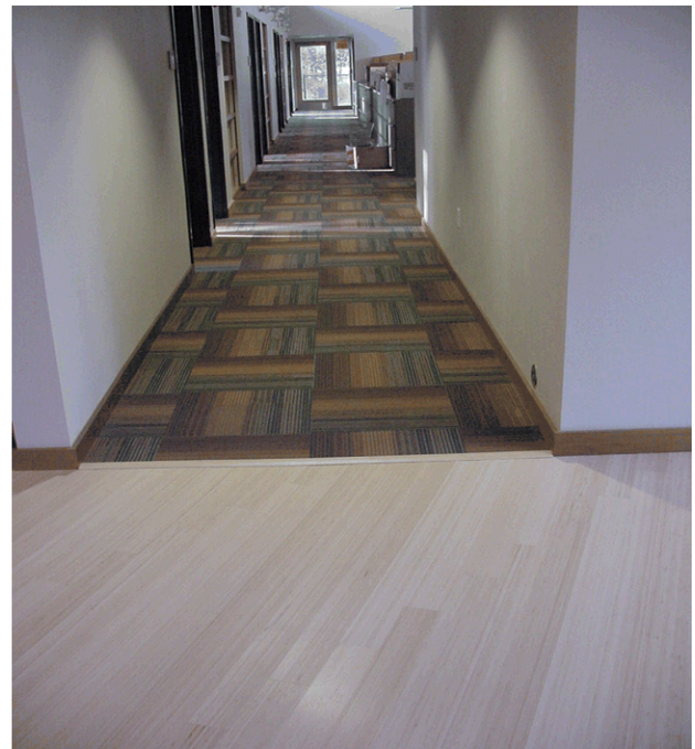
Herbert H. Bateman Educational and Admin. Center Bamboo floors and recycled carpet
