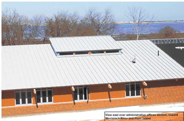
East View Over Admin. Offices
