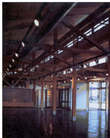
This new building features mechanically operable windows, cool metal roofs, light-control sensors, and structural insulated panels to reduce energy consumption
