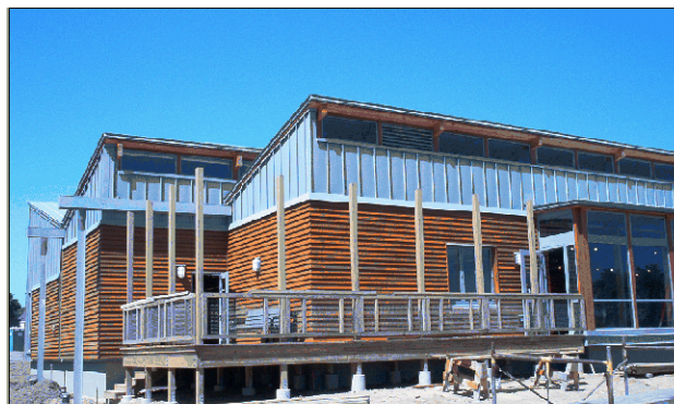
Southeast Corner Viewing Deck
