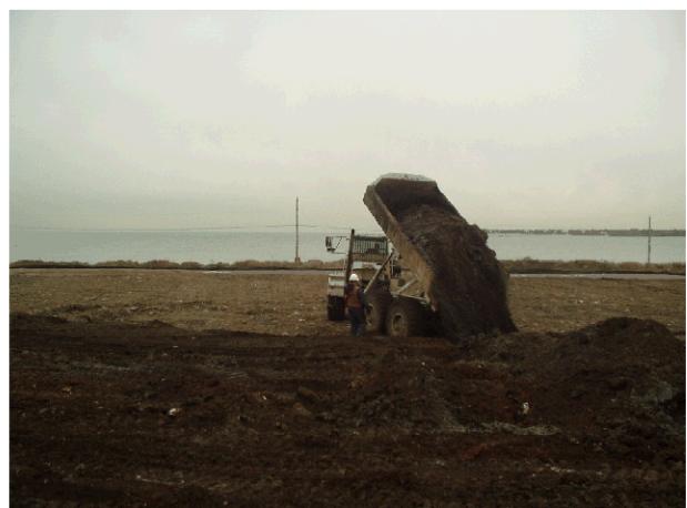
Depositing Soil From Low Fill to High Fill Area
