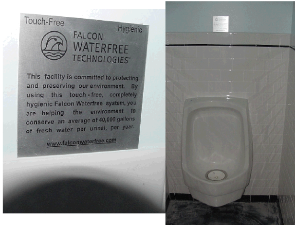
Close-up Sign Above Urinal
