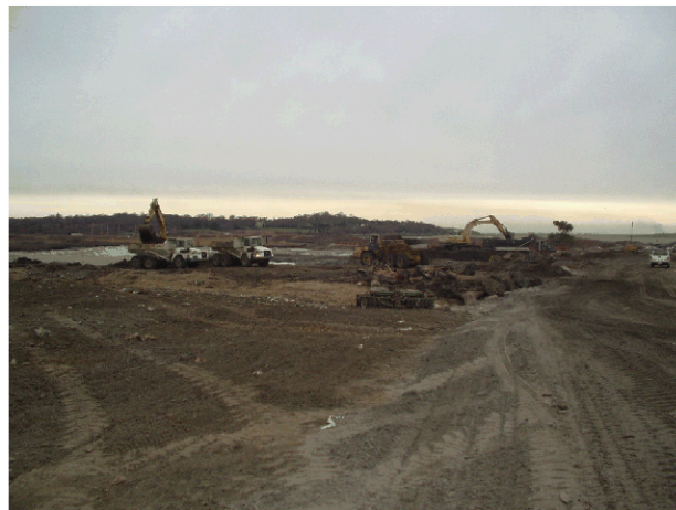
Excavation of Materials in Low Fill Area
