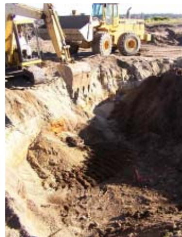
Klamath Marsh NWR - Tank Excavation
