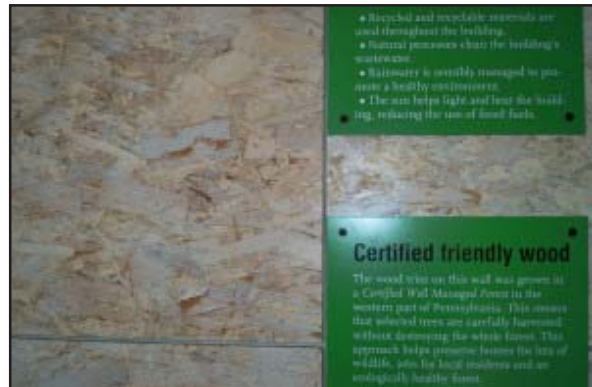
This material used throughout the building is a formaldehyde-free MDF board, produced from waste wood fiber
