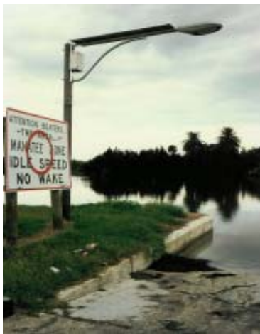
Solar light over a boater safety and manatee warning sign at a remote boat launch site at Merritt Island NWR
