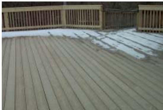
Recycled Plastic Decking at the Boyer Chute NWR, Nebraska
