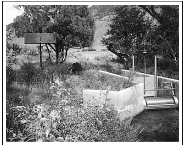
Reese Creek fish trap. NPS photo.
