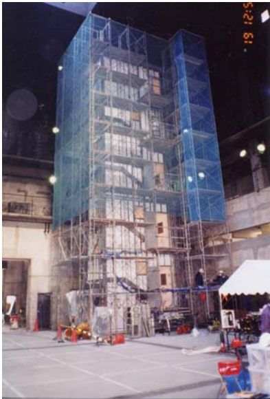
A 4-story mock-up of a staircase.
