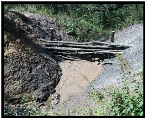
2003 Earth Day Project Construction of Log & Pole Sediment Control Structures on AML Sites Noble County
