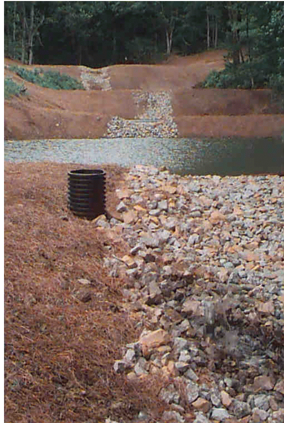
Completed SAPS at Rock Run
