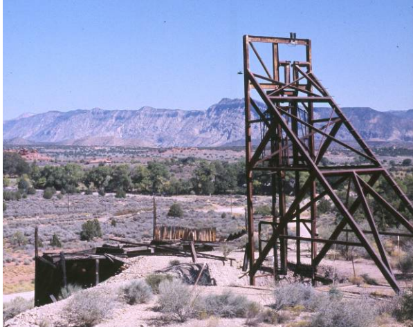
Vertical opening PV2 under headframe at Silver Reef project – 9/27/94
