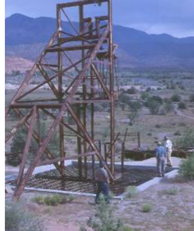
PV2 rebar grate closure at Silver Reef project - 5/11/04
