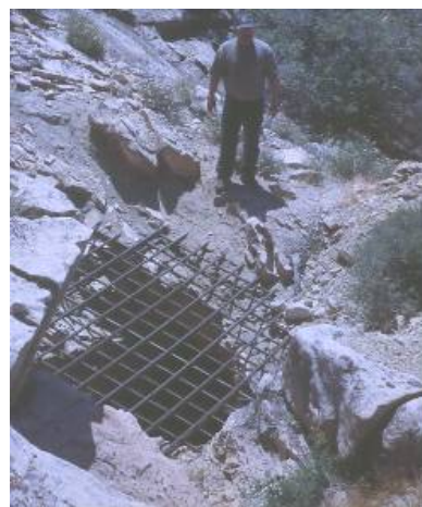
WV50A rebar grate closure at Silver Reef - 5/11/04
