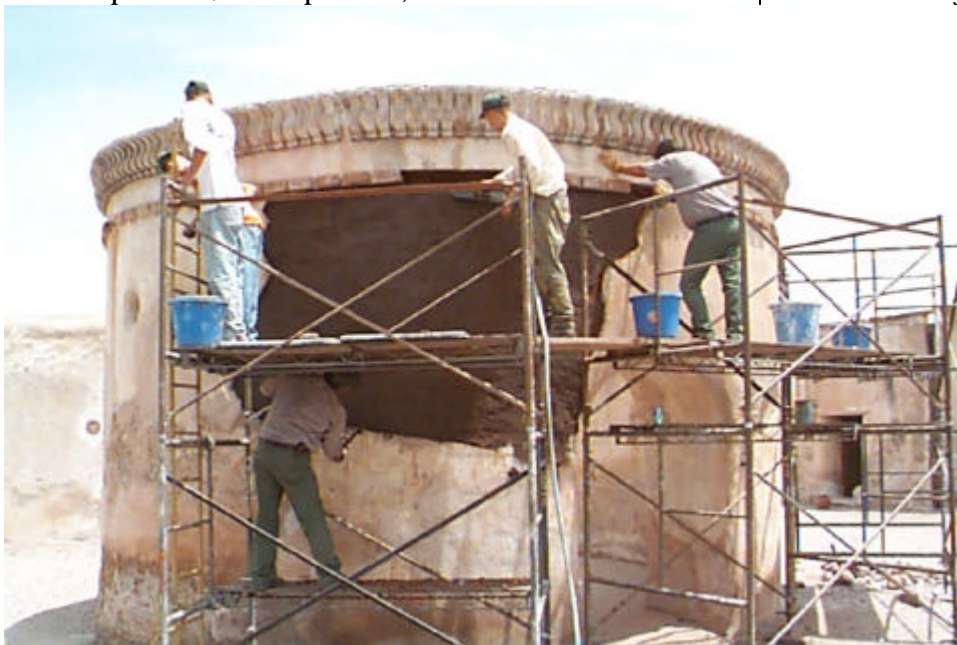
Tumacacori Preservation Crew Repairing Adobe, Tumacacori National Historical Park, AZ.
