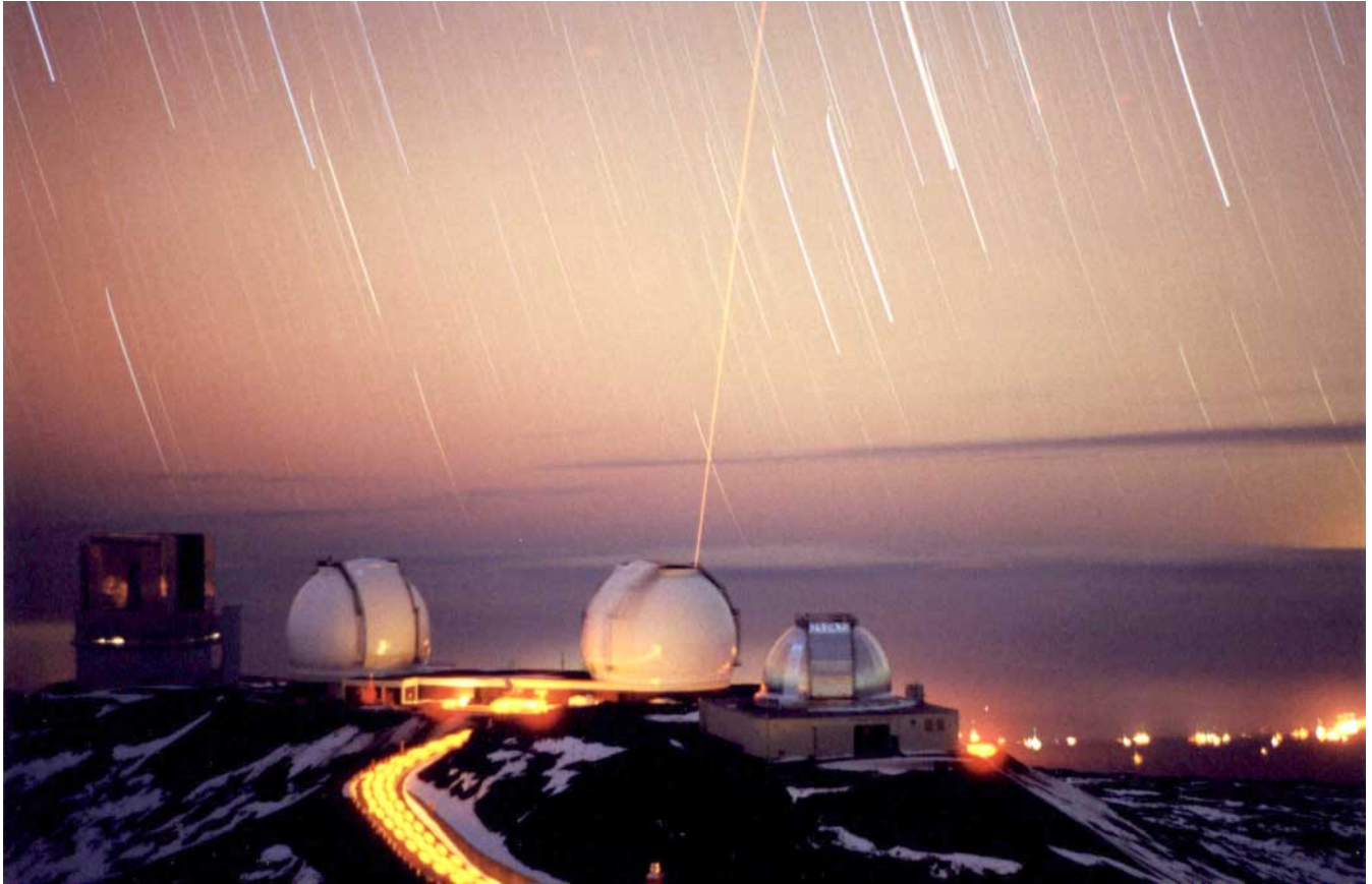
Photo of the Keck “virtual” guide star, showing LLNL-built orange laser beam emerging from the dome of the Keck II Telescope atop 14,000-ft. Mauna Kea volcano in Hawaii. (Photo by John McDonald, Canada-France-Hawaii Telescope Corp.)
