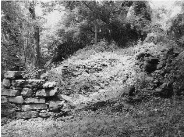
Foundation ruins of the possible block-house. NPS photo.
