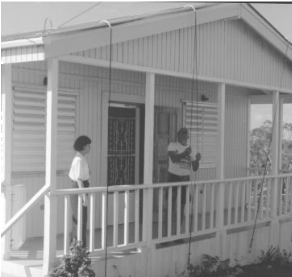
The hurricane straps in this house in Viegies should keep it safe from future storms.
