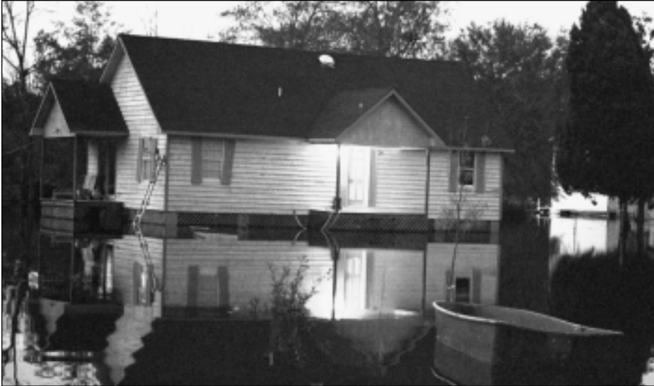
This house was saved from major damage because it was elevated out of harm's way.
