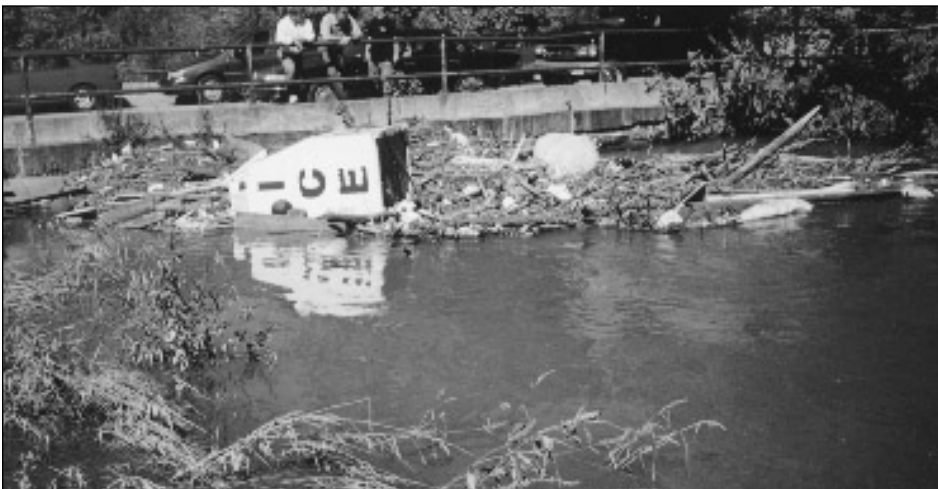
Debris from flooding caused by Tropical Storm Floyd backs up against the West Road Bridge in Danbury.
