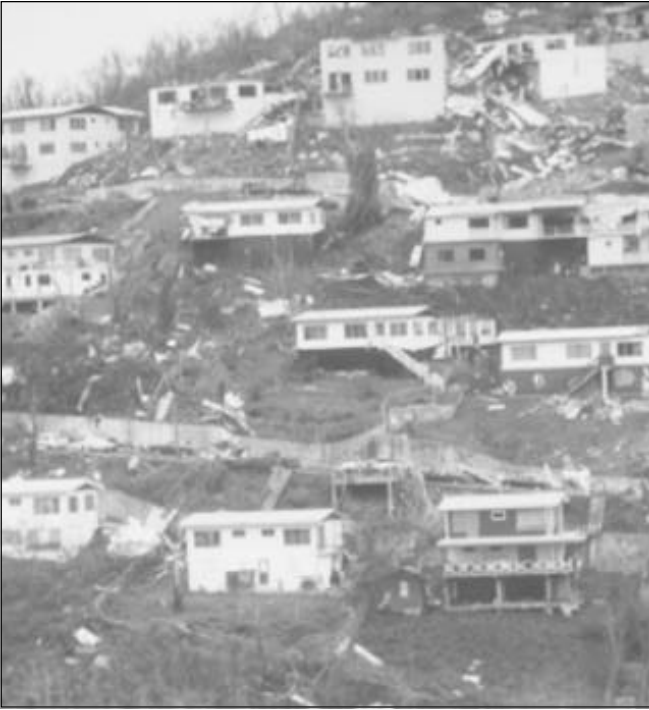
The destructive force of hurricane winds is evident in the damage to these homes in St. Thomas.
