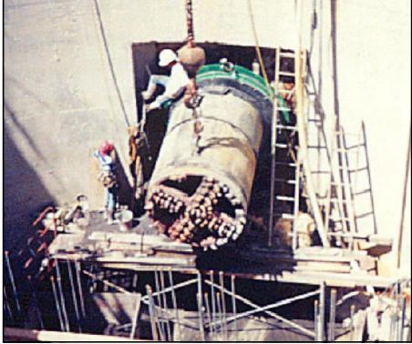
Workers retrieve a tunnel boring machine (TBM) used to excavate an underground passage for a transmission line. TBMs allow water systems to bore through rock at rates faster than conventional drilling and blasting methods. By avoiding the need to tear up streets and set underground explosives, TBMs also minimize traffic disruption and noise for the surrounding areas.
