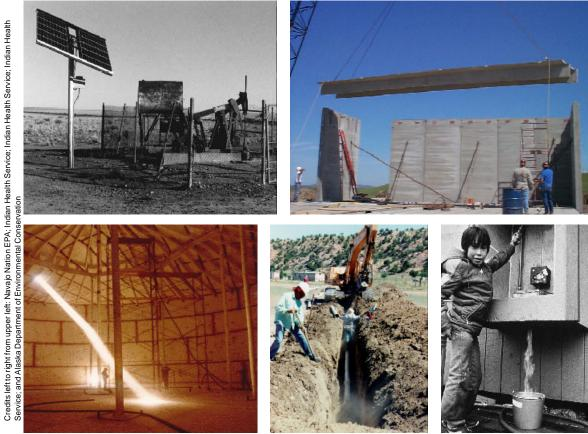
Pictured left to right from upper left: ground water supply, building a new treatment plant, building a ground-level storage tank, laying distribution mains, and collecting drinking water from a watering point.
