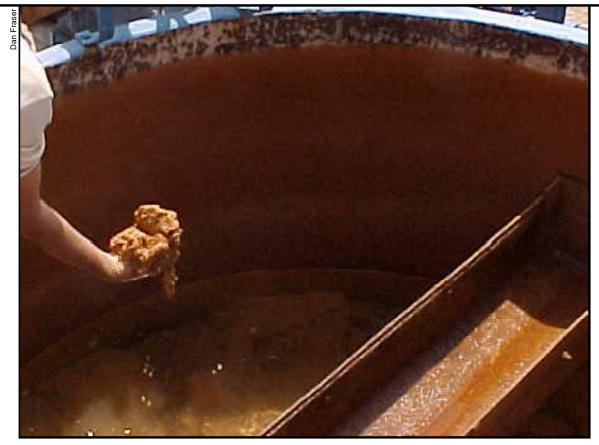
Filtration plants consist of a series of treatment stages, each of which is critical to the production of safe water. Shown is a filter bed that is clogged with mud and treatment chemicals. The clarifier that should have removed these particulates in the preceding stage is in poor condition and needs to be replaced.
