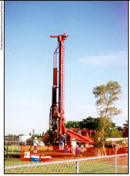
The wells serving the city of Hollywood, Florida, had severe microbiological contamination which fouled the membrane treatment system. In addition, the combined output of the wells could not meet demand and the distribution system routinely failed to reach minimum pressure standards. With a \$13 million DWSRF loan, the city drilled 12 new wells and added 1.5 miles of raw water lines.
