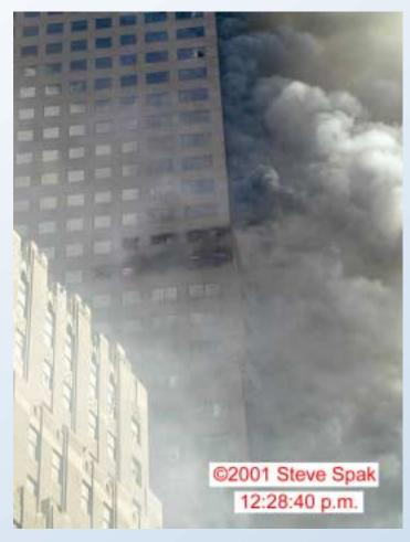
Fires in WTC 7—which began soon after WTC 1 collapsed—were observed on Floors 7, 8, 9, and 11 near the middle about half an hour before collapse; Floor 12 was burned out by this time. Fires were also seen on Floors 12, 13, 22, 29, and 30 at various times during the day.
