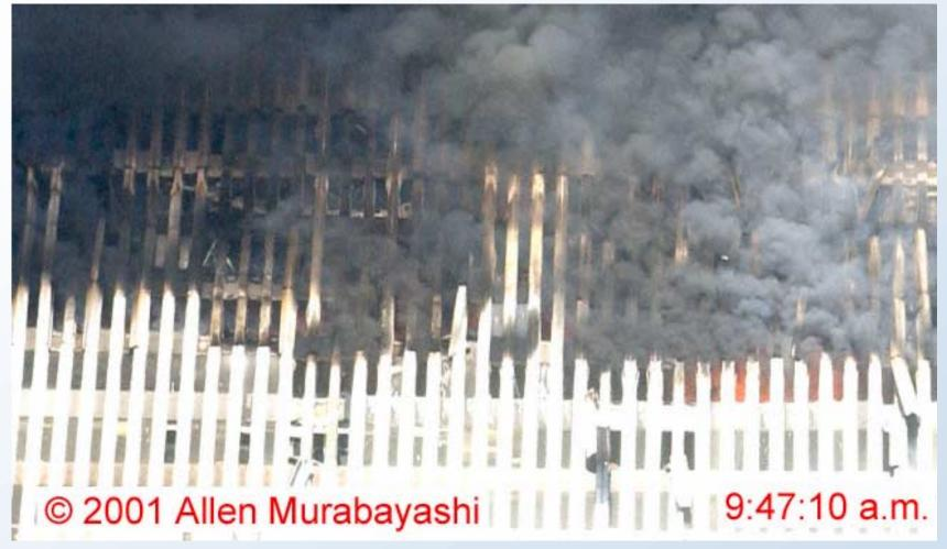
East Face of the South Tower. Image shows what appear to be a floor slab from the 83rd floor hanging across window opening over a large fraction of the 82nd floor.
