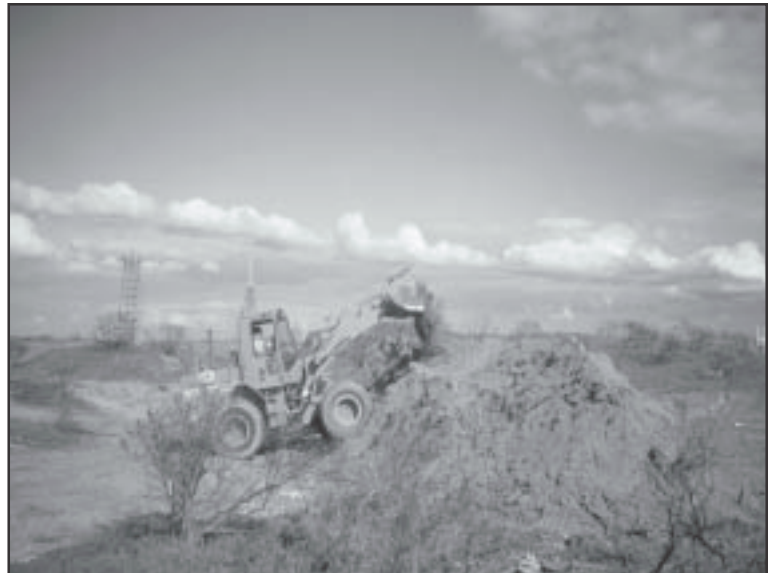
Constructing dunes using existing sand.
