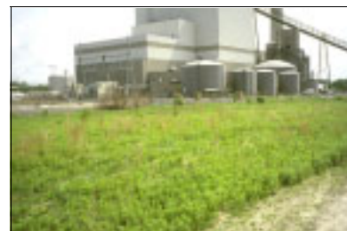
Restored native vegetation near Logan Generating Plant.
